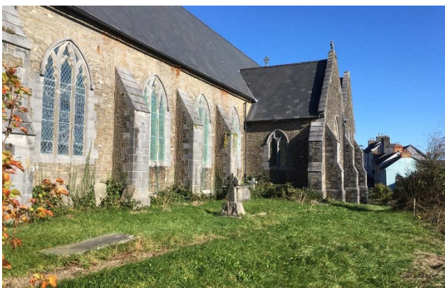
Above : South side of the church showing nave (left) and south chapel (centre right).
