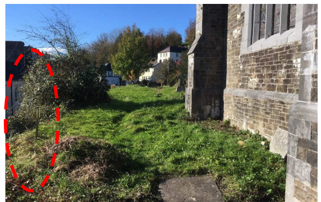
Above : South side of South Chapel. Guarding needed to protect people from falling off the churchyard retaining wall (left of picture).
